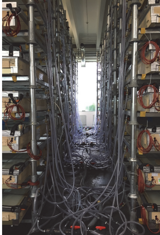
Figure 17: ETFE-modules with temporary air supply for their transportation, ©Taiyo Europe
